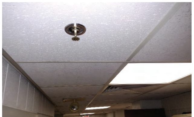
FRP 3 – Typical Semi-Recessed Sprinkler Head
