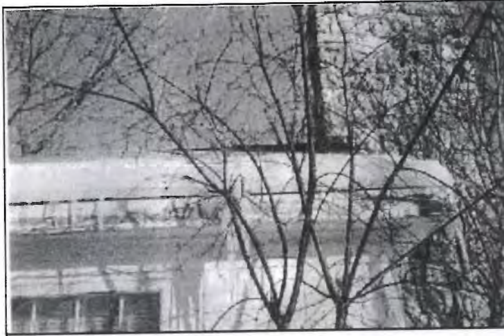
Photo No. 11 Roof and Gutter - Addition Stone School
