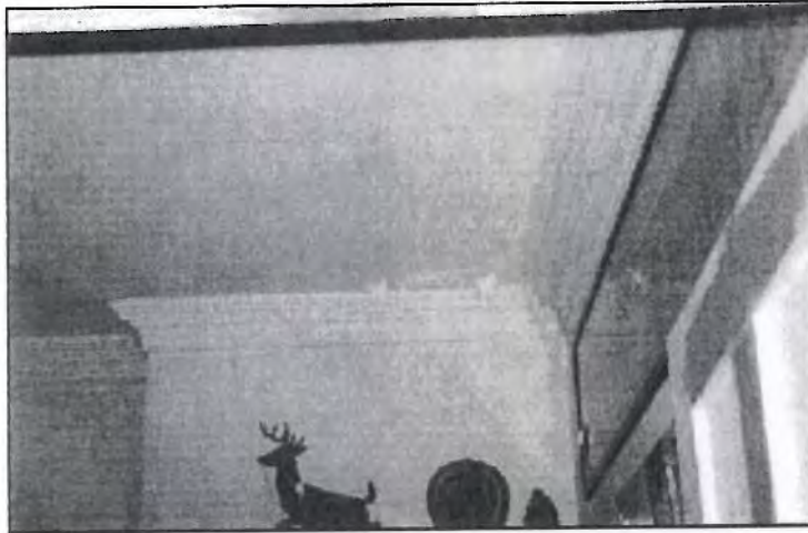
Photo No.9 Dining room Ceiling Stone School
