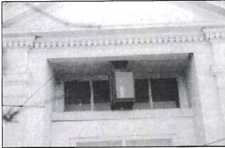
Photo No. 5 Front Door Transom Stone School
