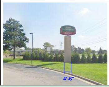
**EXISTING CABINET & POLE COVER TO BE REMOVED; NEW POLE COVER AND CABINET TO BE INSTALLED** 7'-0" X 11'-3" PYLON SIGN
