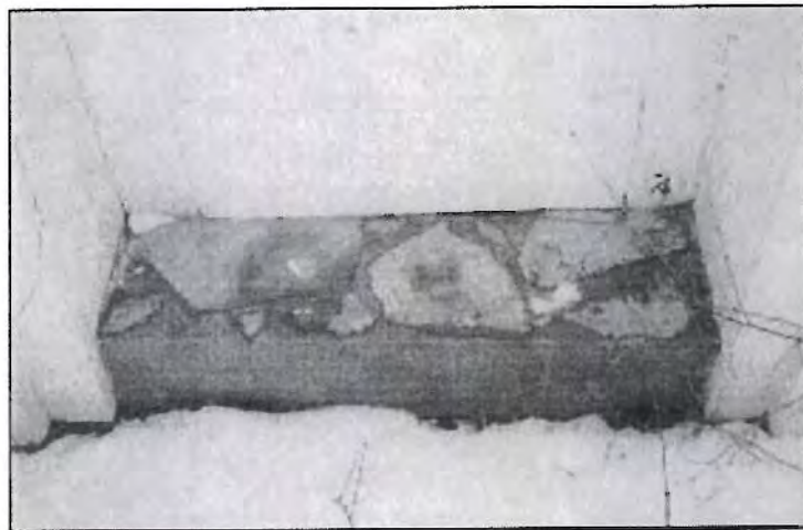
Photo No. 6 Stone Door Sill Stone School
