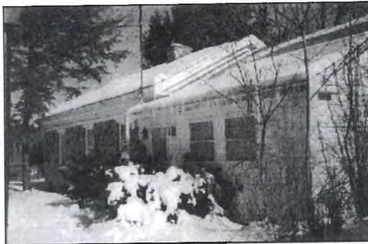
Photo No. 12 Addition Stone School
