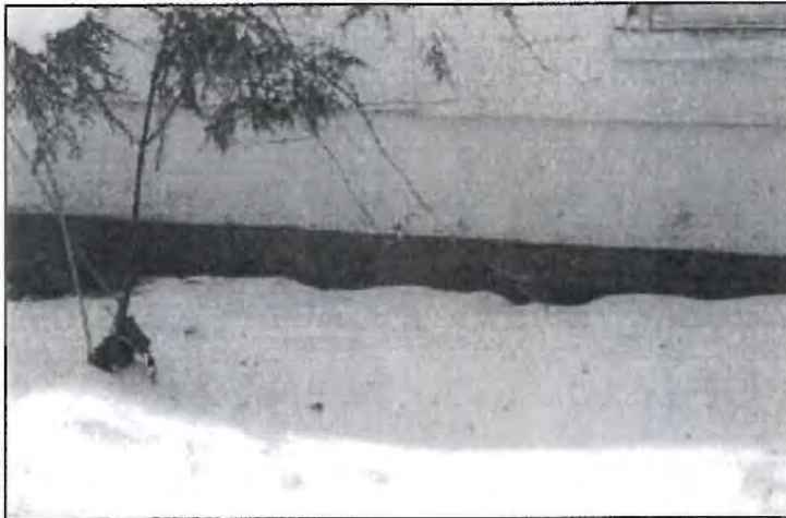
Photo No. 19 Addition Foundation Stone School
