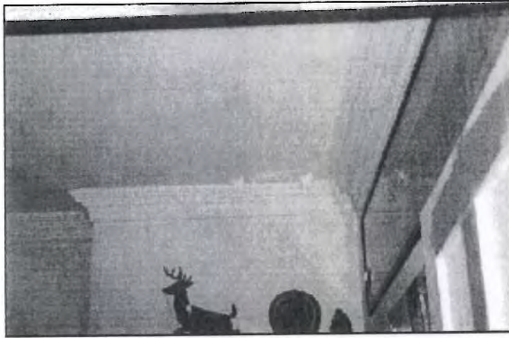
Photo No.9 Dining room Ceiling Stone School
