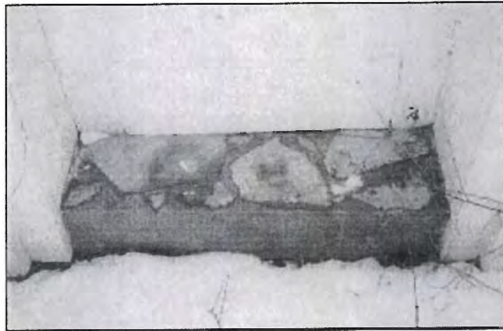
Photo No. 6 Stone Door Sill Stone School
