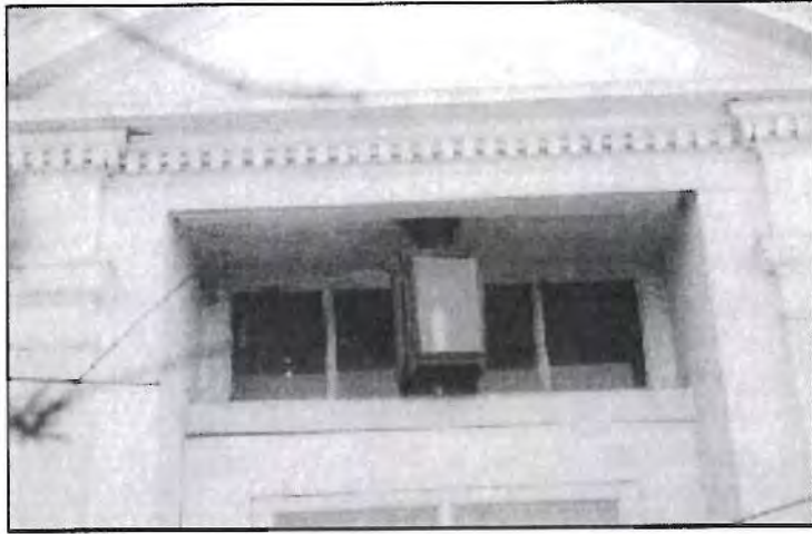
Photo No. 5 Front Door Transom Stone School
