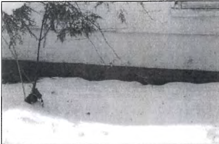
Photo No. 19 Addition Foundation Stone School
