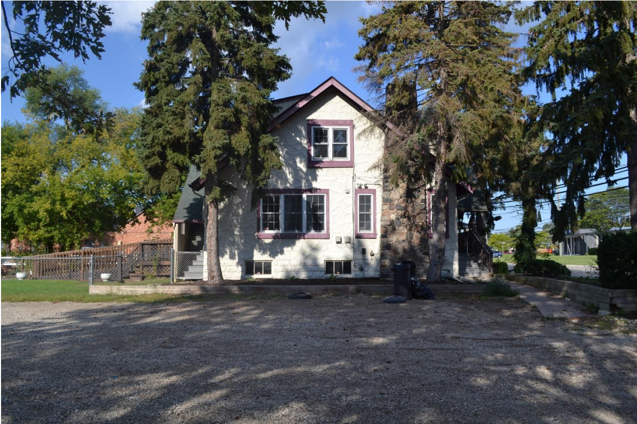
East elevation, image taken facing west - 09-08-21
