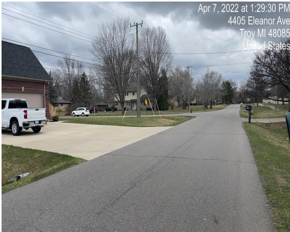
Photograph No. 6: Eleanor Drive - Heading South Date: 04/7/2022 Photographer: Richard Boateng & Genevieve Schneemann
