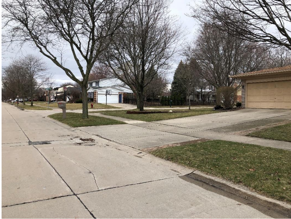
Photograph No. 5: Oakcrest Drive - Heading West and looking right Date: 03/24/2022 Photographer: Richard Boateng & Genevieve Schneemann
