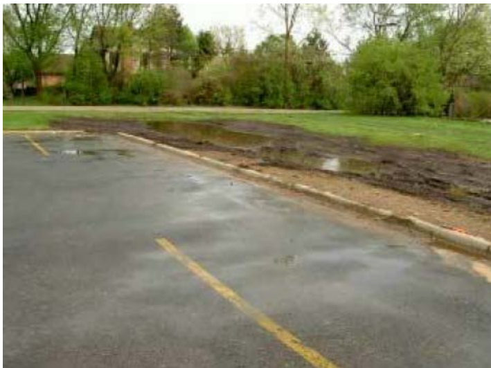
Beach Road Park, pre-construction.
