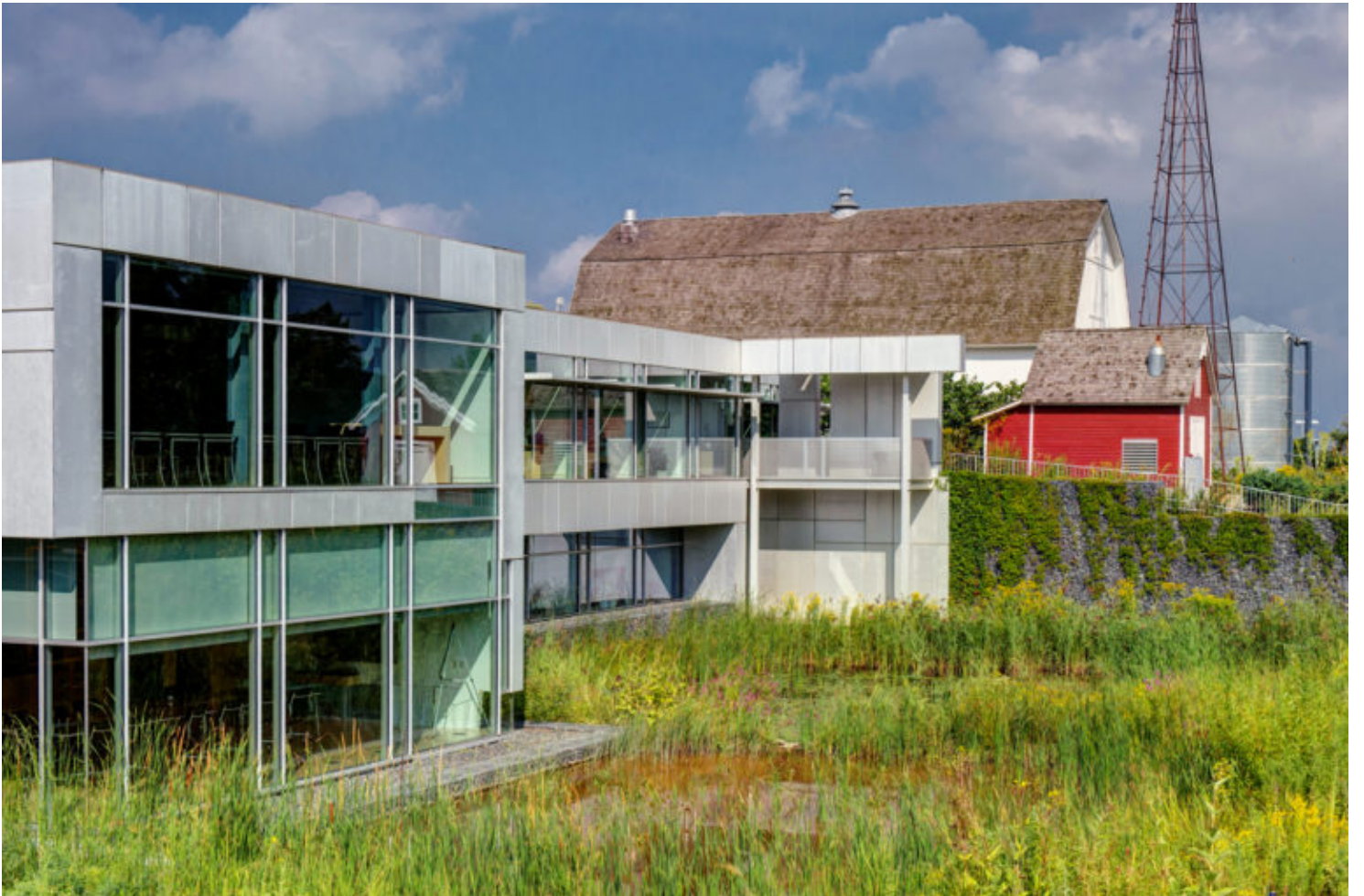
The Kresge Foundation headquarters
