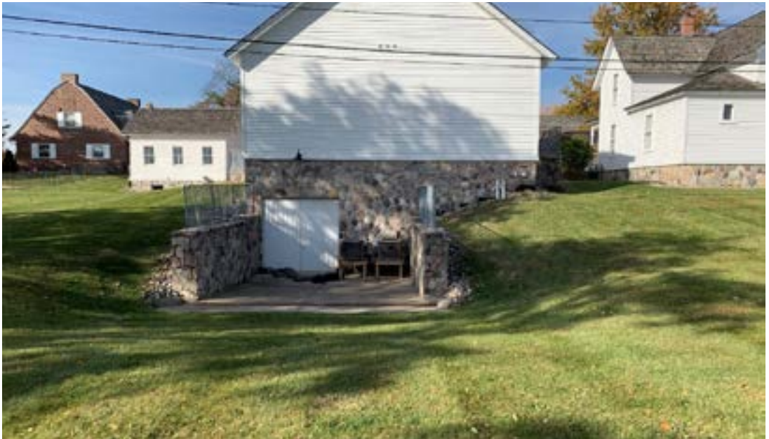
A westward perspective of the grading challenges behind the Church.
