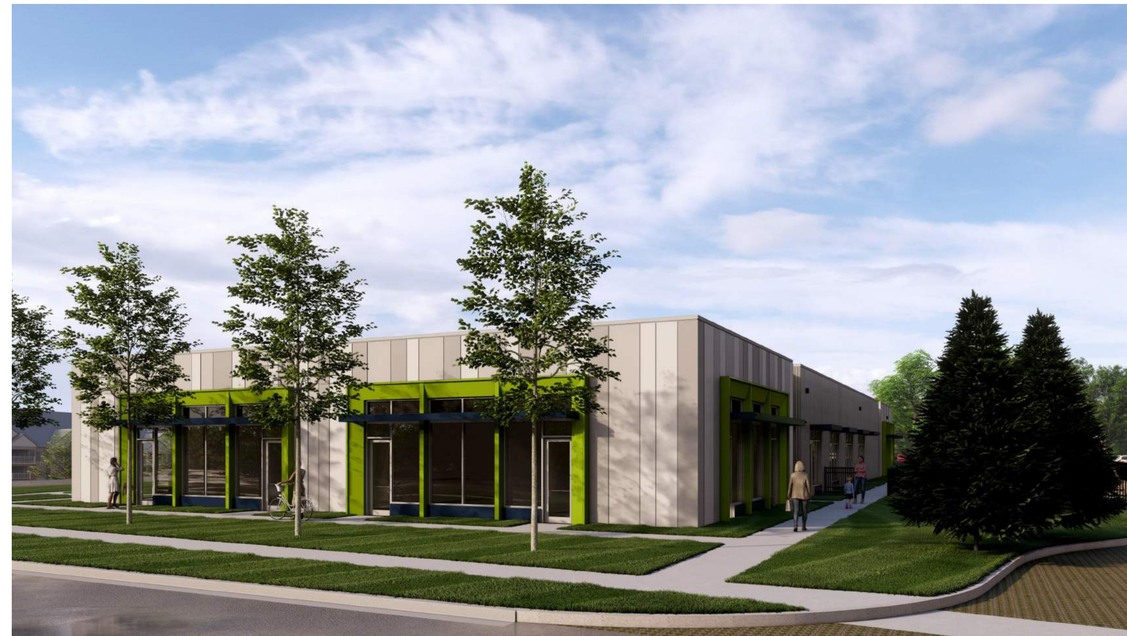
View of side facade from Crooks Rd.
