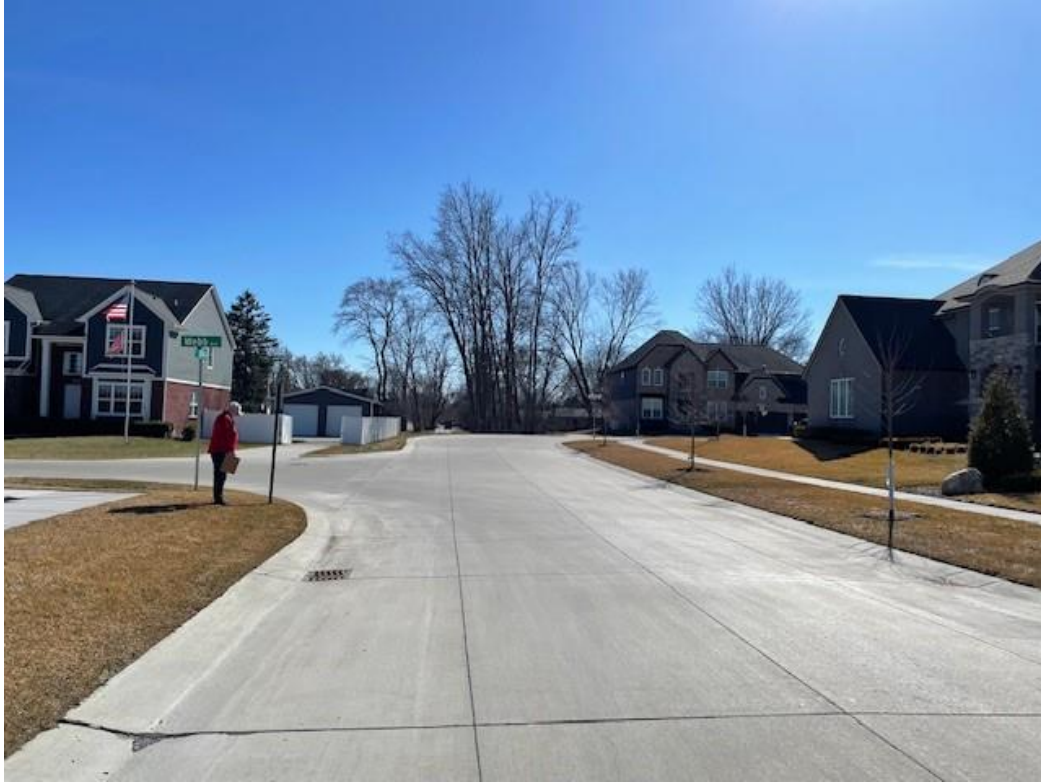
Photograph No. 7: Virgilia Dr - Heading South Date: 02/29/2024 Photographer: Lauren Hull
