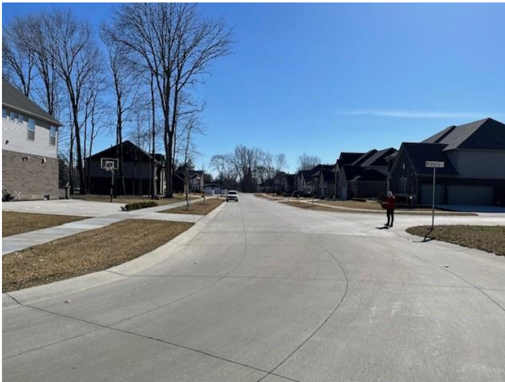
Photograph No. 6: Virgilia Dr - Heading South Date: 02/29/2024 Photographer: Lauren Hull
