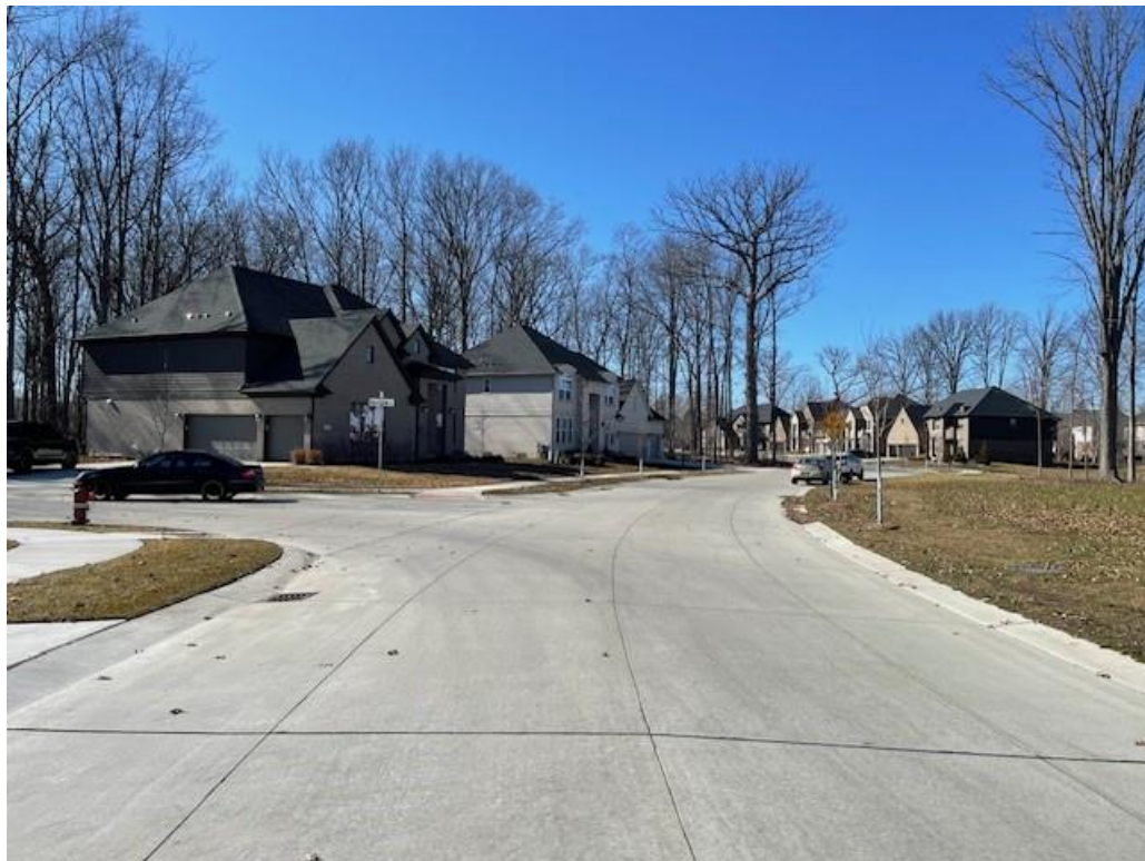
Photograph No. 2: Blakely Ct - Heading West Date: 02/29/2024 Photographer: Lauren Hull
