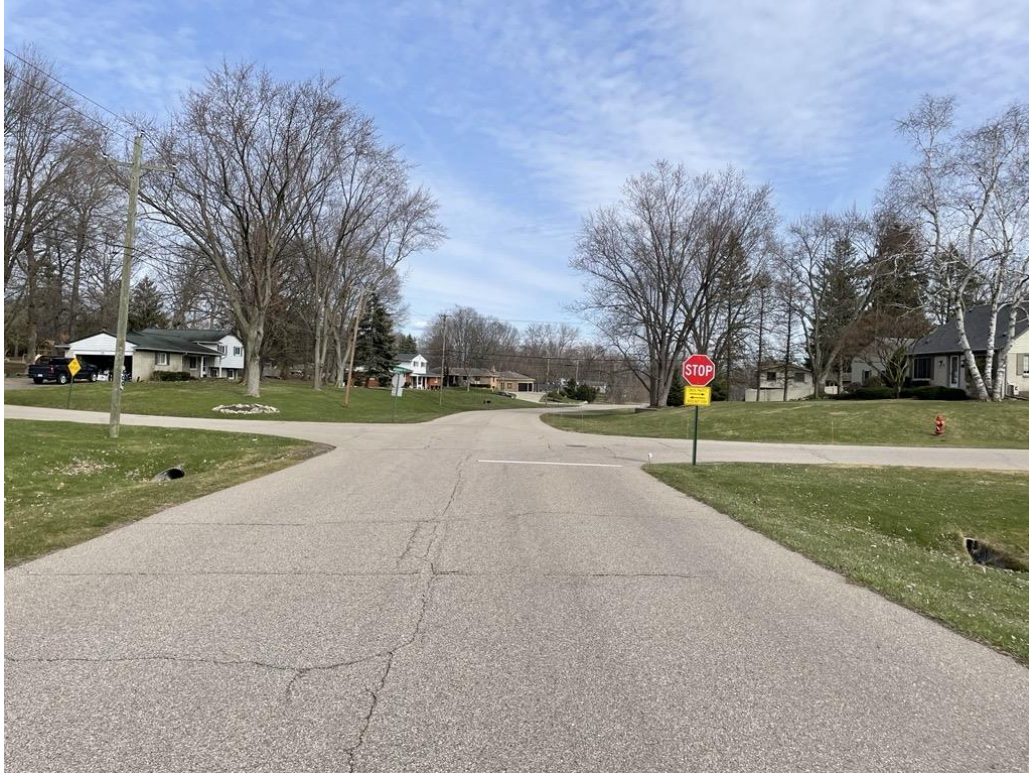
Photograph No. 5: Troyvally Drive – Heading East Date: 03/21/2024 Photographer: Lauren Hull
