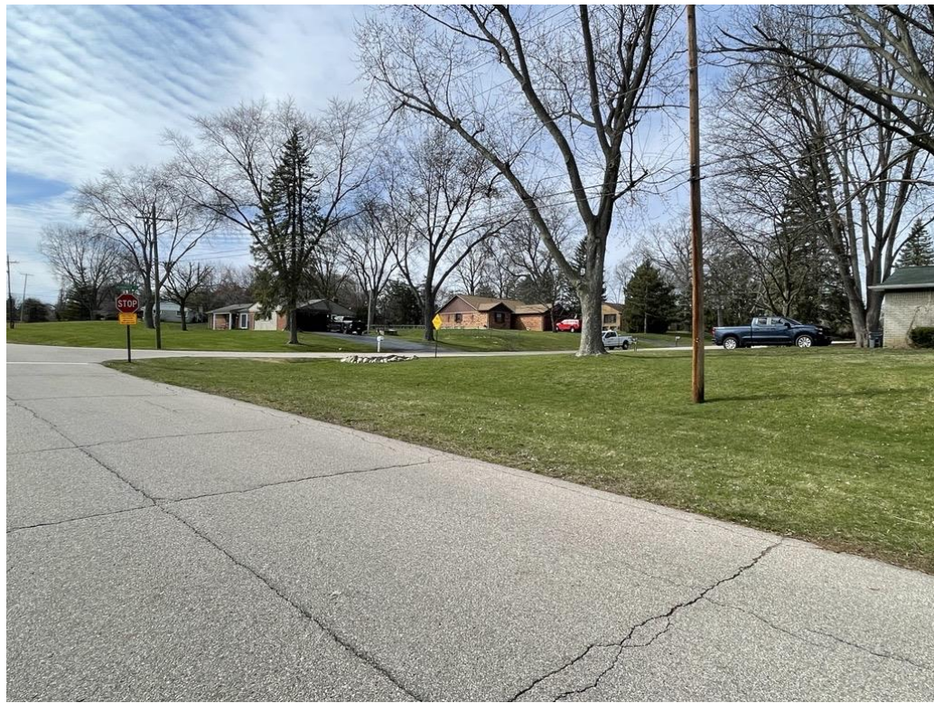
Photograph No. 12: Troyvally Drive - Heading West Looking Right Date: 03/21/2024 Photographer: Lauren Hull
