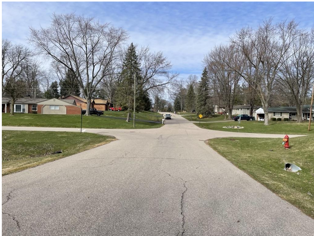
Photograph No. 2: Herbmoor Drive - Heading North Date: 03/21/2024 Photographer: Lauren Hull
