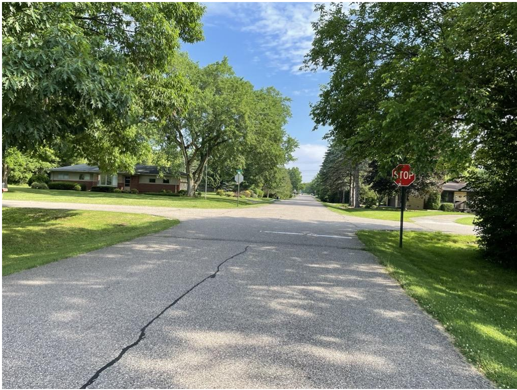
Photograph No. 2: Donaldson Road - Heading North Date: 06/18/2024 Photographer: Lauren Hull
