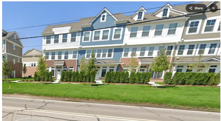
Row of arborvitae between building and ROW
