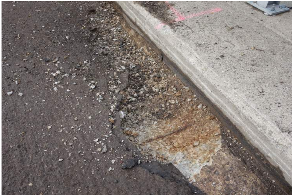
Top Flange of Box Beam Deterioration
