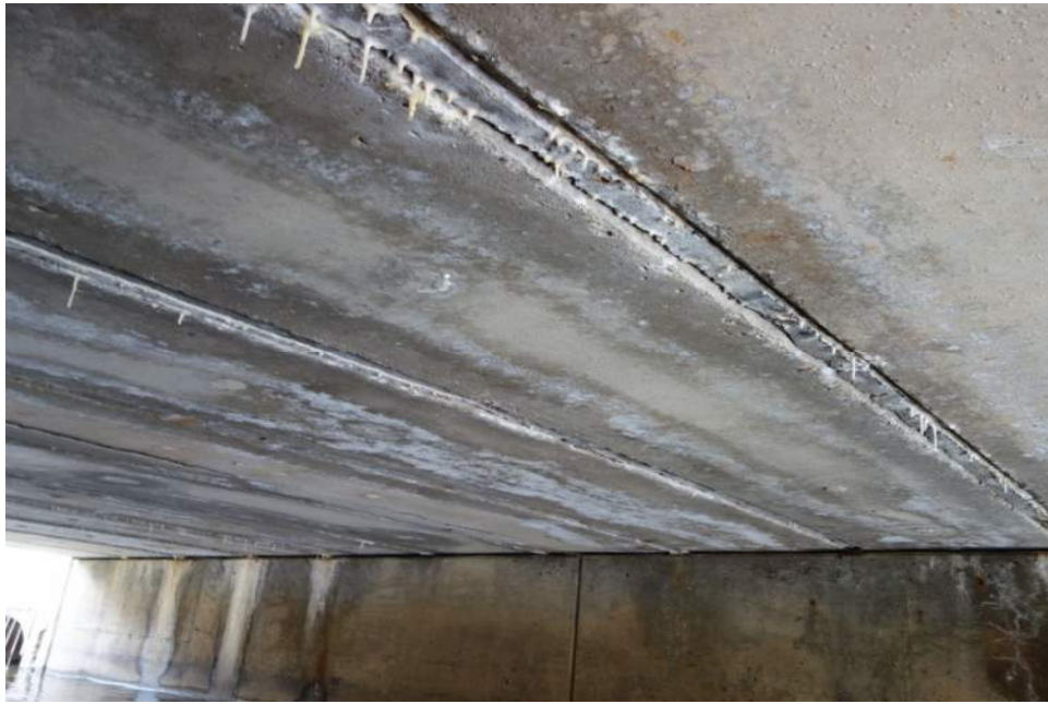
Typical Leaching Joint Between Box Beams
