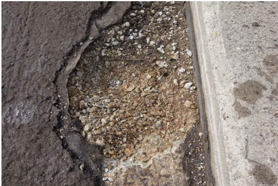
Top Flange of Box Beam Deterioration
