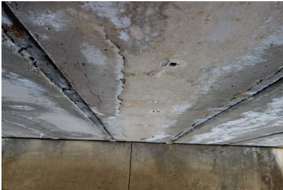
Beam 5W Cracking
