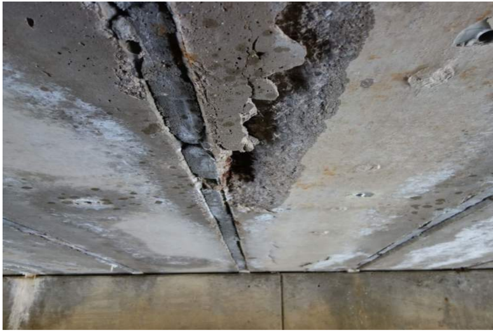
Beam 7W Delamination and Broken Strand
