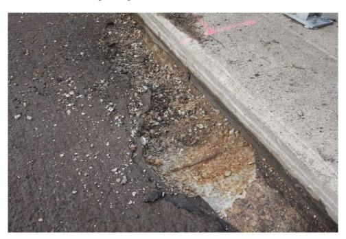
Top Flange of Box Beam Deterioration
