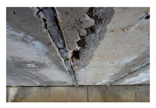
Beam 7W Delamination and Broken Strand
