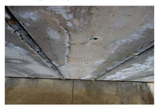
Beam 5W Cracking
