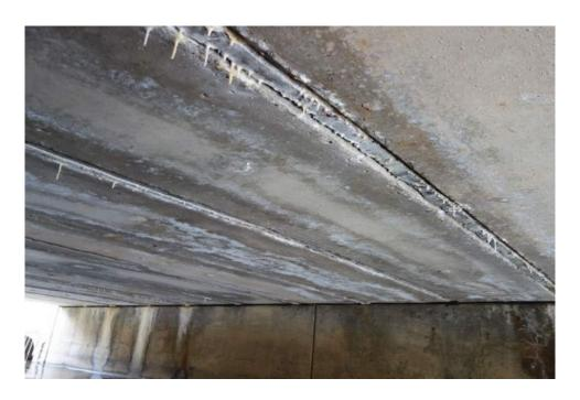
Typical Leaching Joint Between Box Beams
