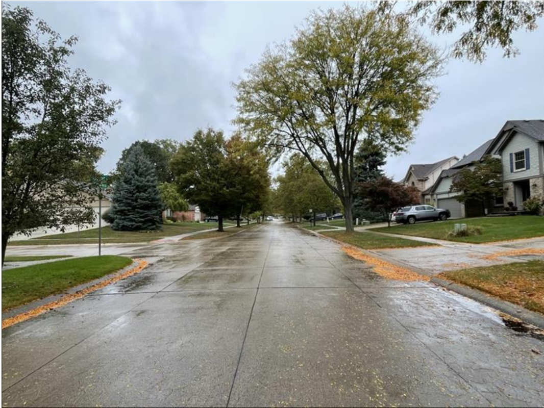
Photograph No. 28: Wayfarer Drive - Heading North Date: 10/07/2025 Photographer: Lauren Hull
