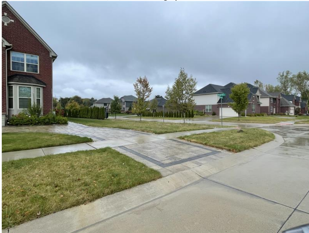
Photograph No. 13: Macaw Drive - Heading North Looking Left Date: 10/07/2025 Photographer: Lauren Hull
