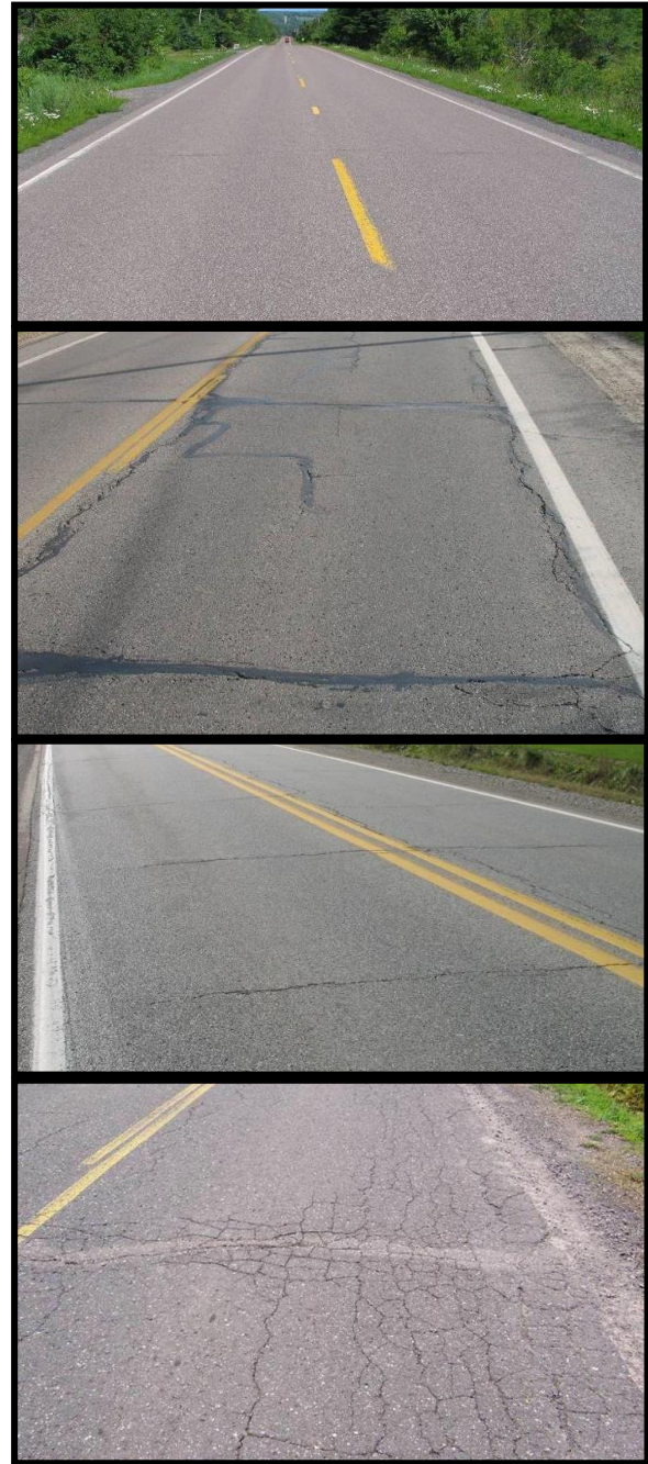
Figure 1: Top image – PASER 8 road that is considered “good” by the TAMC exhibit only minor defects. Second image – PASER 5 road that is considered “fair” by the TAMC. Exhibiting structural soundness but could benefit from CPM. Third image – PASER 6 road that is considered “fair” by the TAMC. Bottom image – PASER 2 road that is considered “poor” by the TAMC exhibiting significant structural distress.
