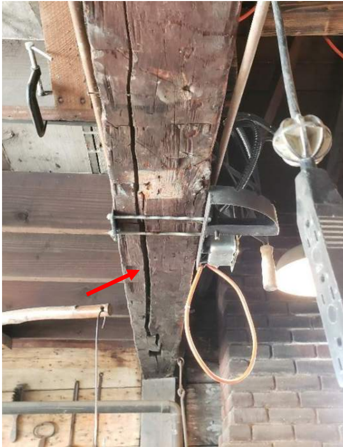
Figure 22. Check on center beam underside.
