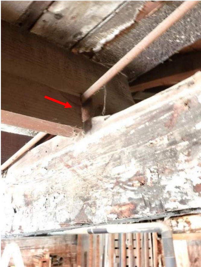
Figure 16. Large notch to accommodate center beam tension rod.
