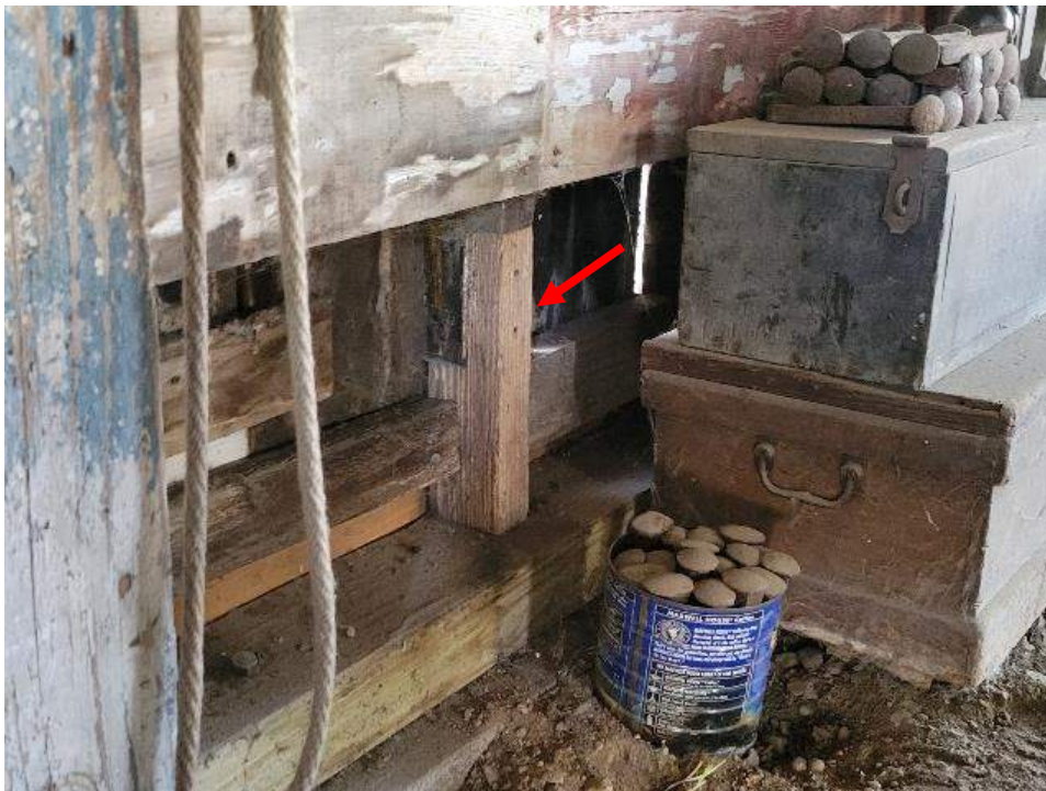
Figure 25. Wood splice at a wall stud.
