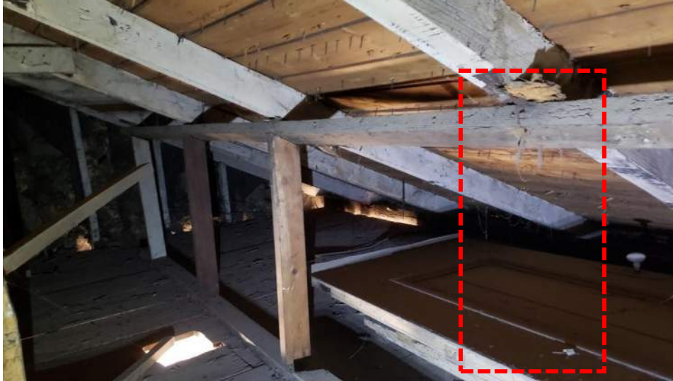
Figure 14. Missing stud below rafter in the west knee wall.
