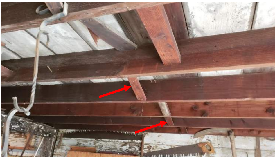
Figure 17. Cross-bridging at the loft floor joists.
