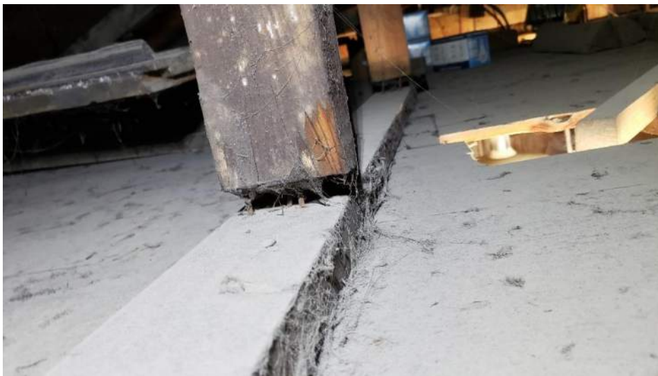
Figure 13. Knee wall stud is not bearing directly on the knee wall bottom plate.
