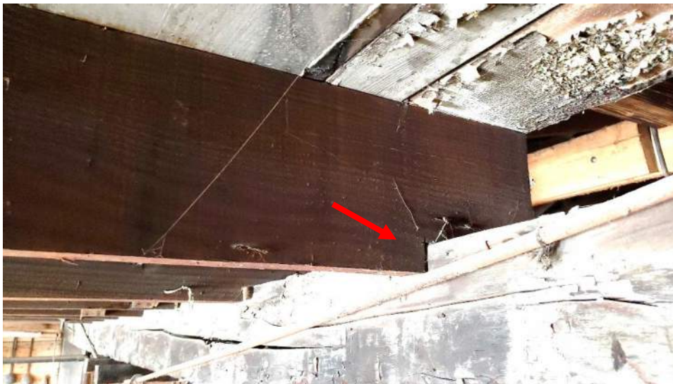
Figure 15. Typical notch in loft area joist bearing end.
