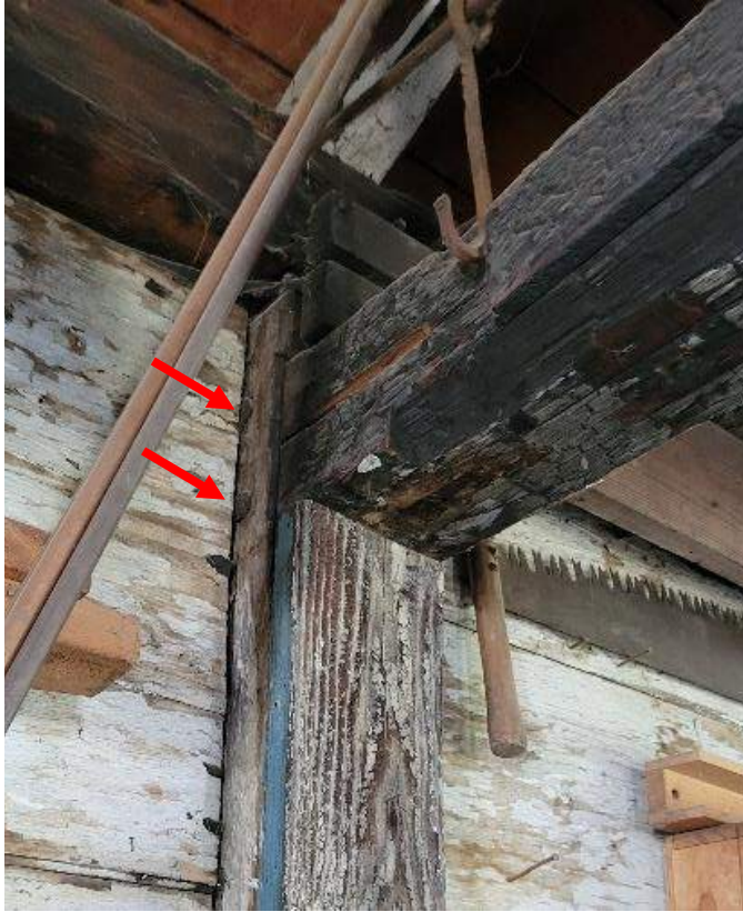
Figure 24. Wood trennels on side of column (arrows).
