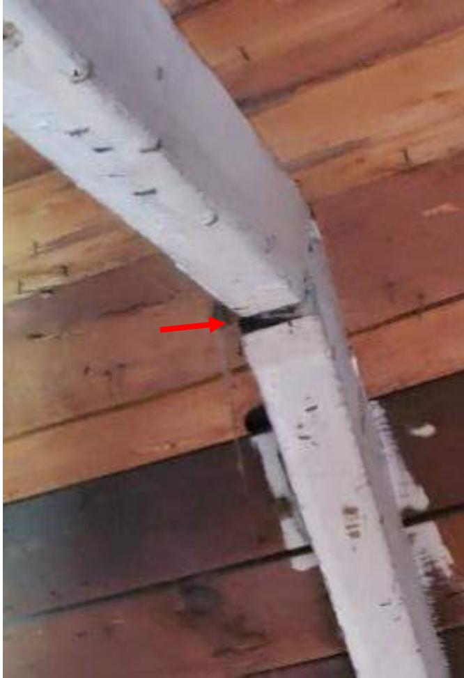
Figure 8. Unpainted end of rafters. Note paint on underside of some of the roof decking.
