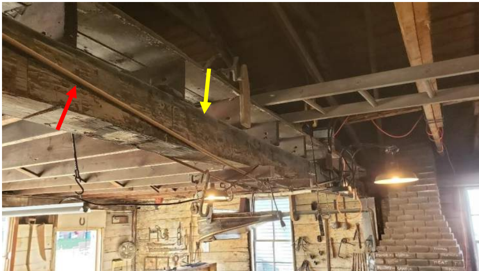
Figure 19. Post-tensioned 'truss' comprised of timber (yellow arrow) and tension rods (red arrow).
