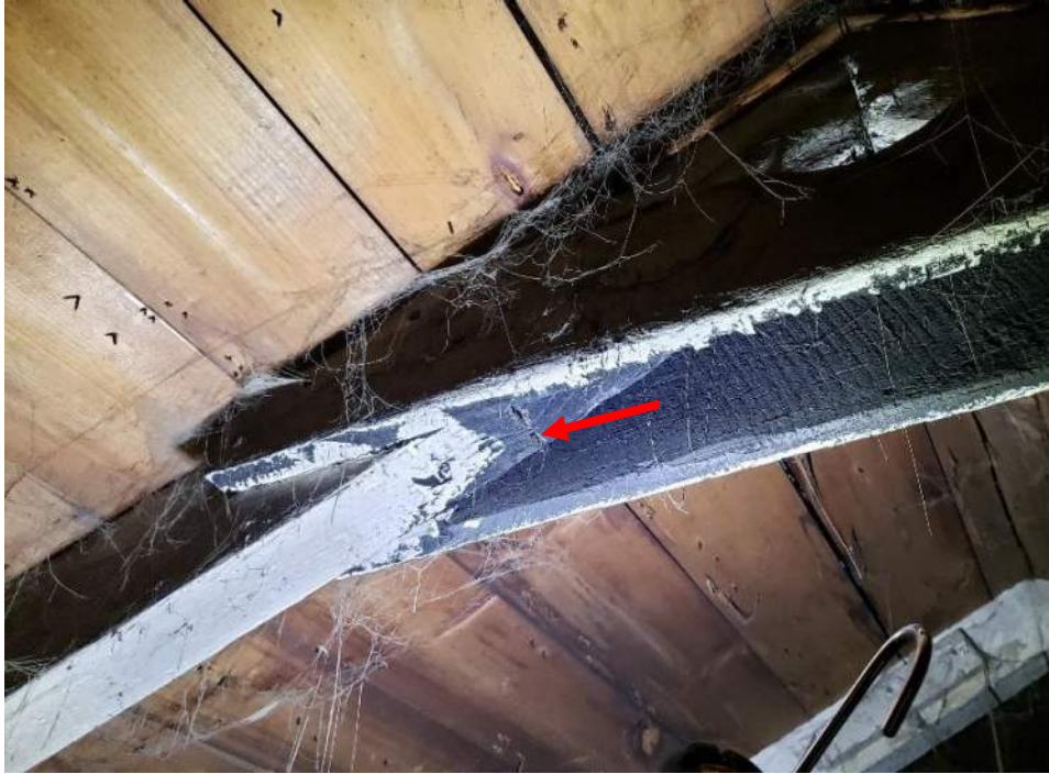
Figure 10. Fractured rafter (arrow) near the ridge, where char is located.
