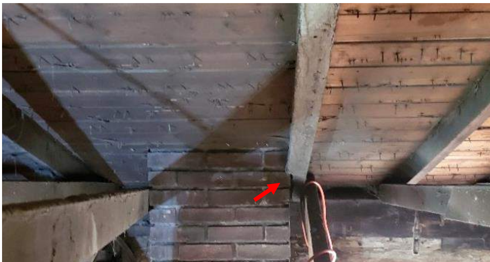
Figure 7. Notched rafter at chimney.
