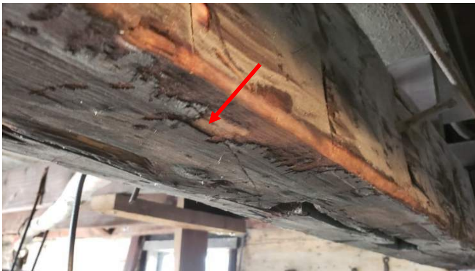
Figure 23. Surface char on center beam underside.
