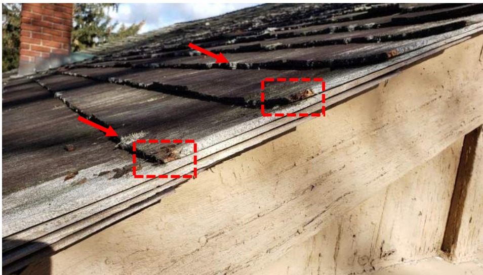
Figure 2. Localized decay (boxed areas) and lichen growth (arrows) on the roof shingles.
