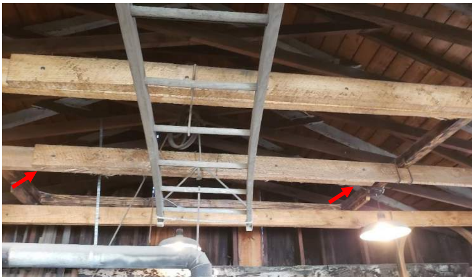
Figure 9. Rafter ties bolted and lapped.
