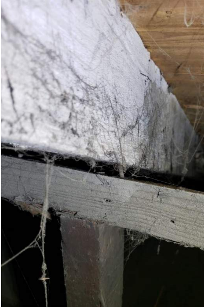
Figure 12. Rafter not bearing directly on a knee wall top plate.
