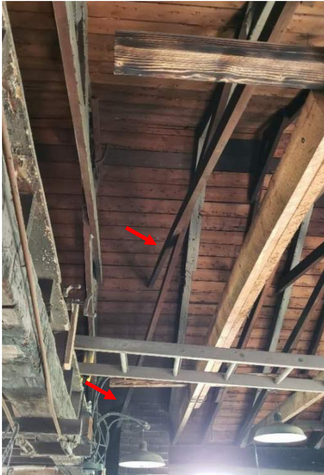
Figure 6. Cross-bracing is unsecured to west rafter to accommodate chimney.
