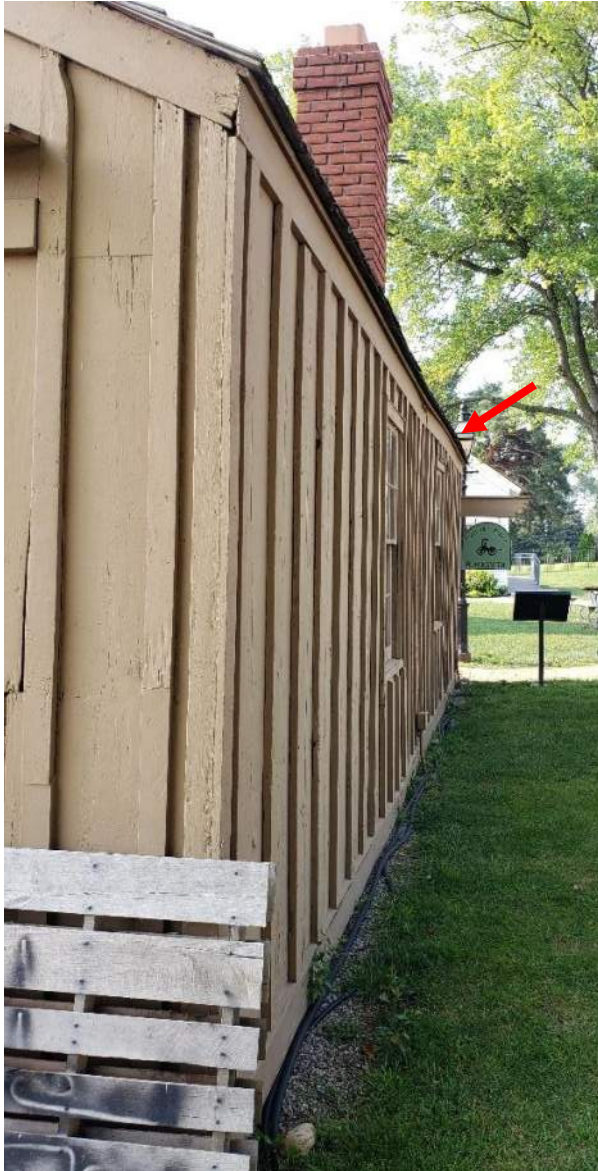
Figure 26. West wall of the building. The arrow indicates the approximate location of maximum outward displacement.
