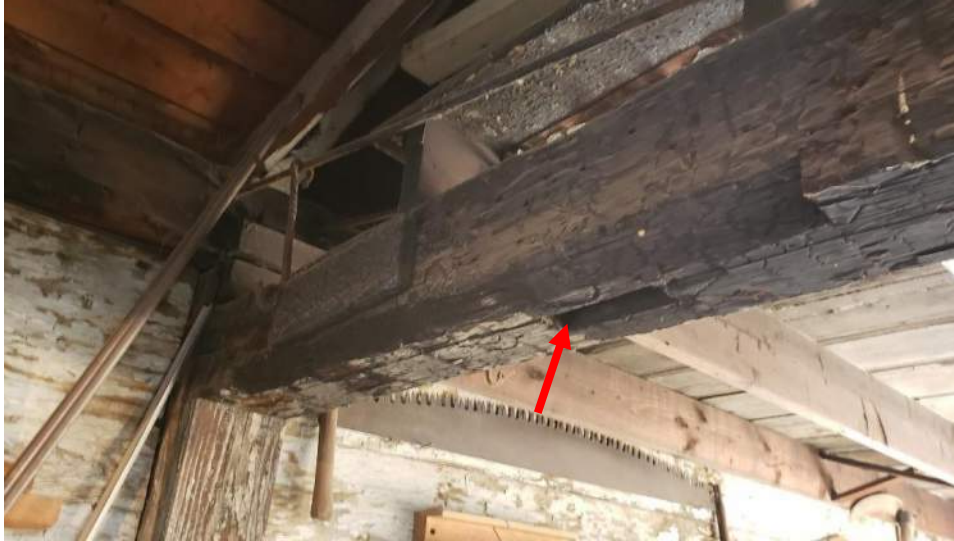
Figure 20. Abandoned mortise on center beam underside.
