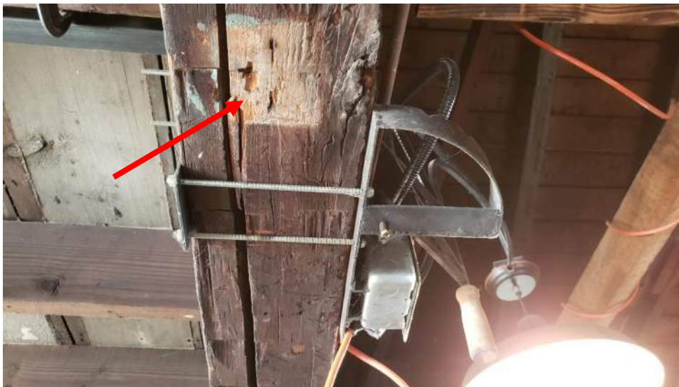
Figure 21. Shadow of likely previous column on underside of center beam.
