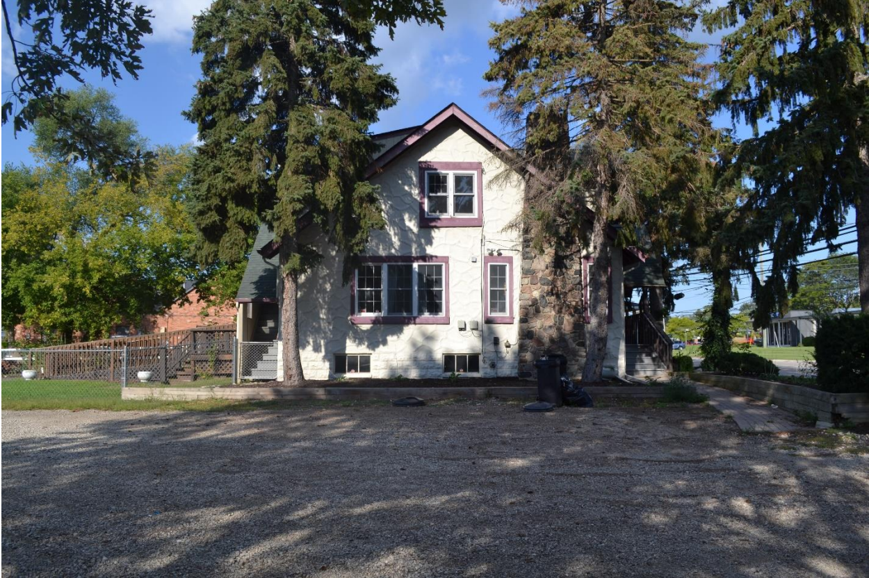
East elevation, image taken facing west - 09-08-21
