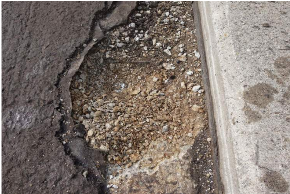
Top Flange of Box Beam Deterioration
