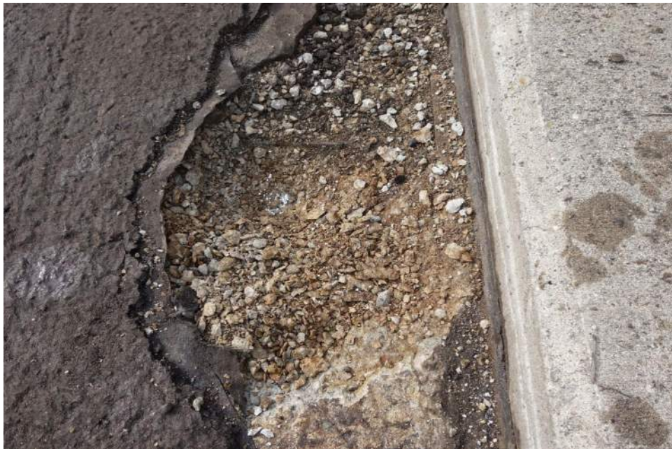
Top Flange of Box Beam Deterioration
